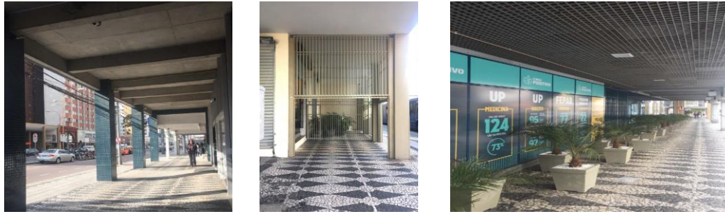
Figure 1. (a) Galleries at Sete de Setembro Avenue, (b) gates closing the galleries, and (c) cement flower pots.
